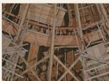
Inspection walkway @ rotundatrust.org.uk CC BY 4.0
