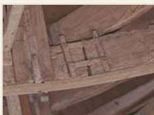
Iron strap connection @ rotundatrust.org.uk CC BY 4.0
