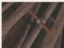
Bracing and sarking @ rotundatrust.org.uk CC BY 4.0
