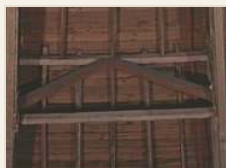
Mid-height bracing @ rotundatrust.org.uk CC BY 4.0
