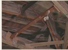
Cross-bracing @ rotundatrust.org.uk CC BY 4.0
